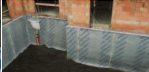
DELTA®-TERRAXX offers permanent-filtration drainage.
